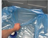
When the liner is half full, pull the four sides towards the centre to unfold the rest of the liner.
